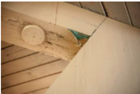
Water damage to interior wooden ceiling and support beams.
