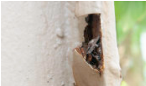
The bell tower is structurally sound but has extensive corrosion and is in need of repair.
