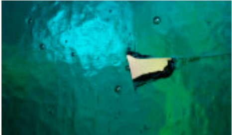
Cracked and missing pieces of stained-glass throughout the church interior need repair or replacement.
