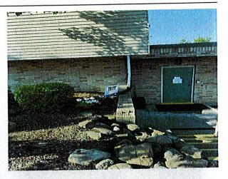
LANDSCAPE RAILROAD TIES – There are landscape railroad ties installed at the north end of the parking lot. Some of them are rotted and deteriorated. It is recommended the deteriorated ties be replaced.
