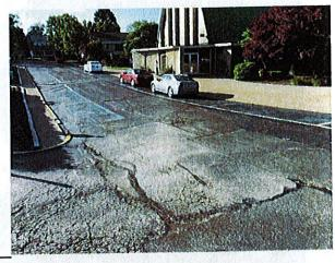
CONCRETE SIDEWALKS AND CURBS – The existing sidewalks and curbs have some good areas and other areas are damaged. Cracks and heaving in the concrete can be tripping safety hazards. It is recommended to replace all damaged concrete sidewalk and curb areas.
